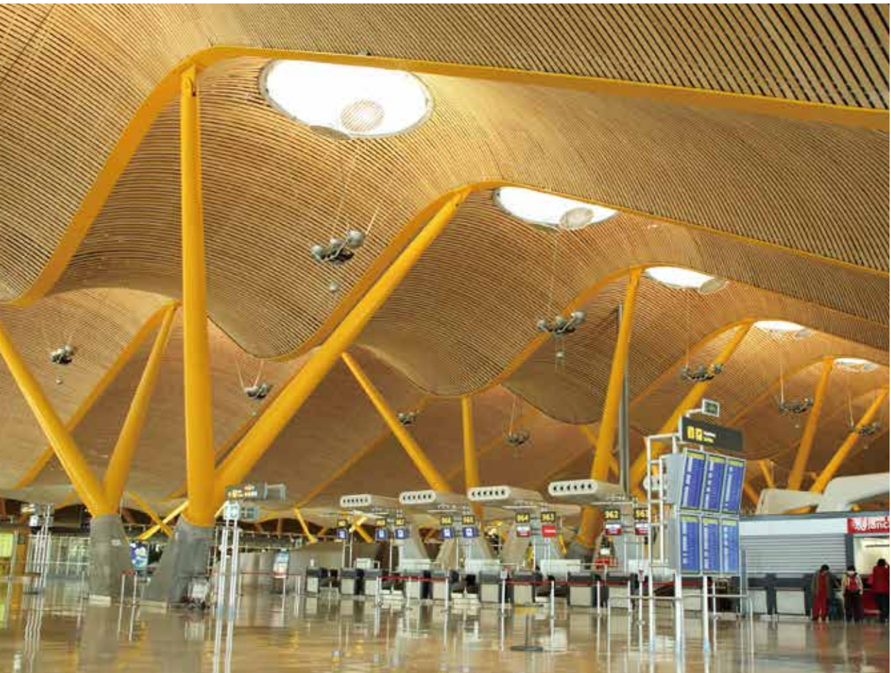
Figure 7. Bamboo is increasingly used by Western architects as building material, for example in the Barajas International Airport in Madrid designed by Richard Rogers.
